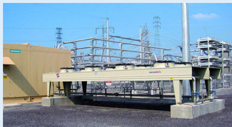
Cheaper, quieter, more compact and more efficient than US products: Güntner drycoolers in a cooling unit built by Anlagenbau Neundörfer for Siemens PTD
