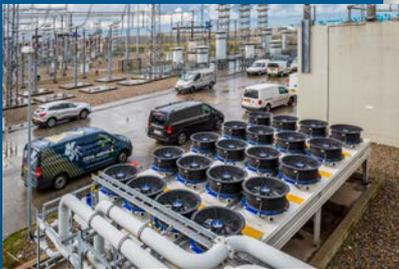
▲ With the help of the new fans from Ziehl-Abegg, power consumption at the converter station in Maasvlakte has been reduced by 450,000 kWh a year and therefore the converter stations' carbon footprint has improved by 51 tonnes of CO<sub>2</sub> equivalent a year.
