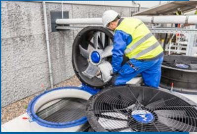
▲ The 40 fans on the Güntner GFH-type FLAT Vario flat bed coolers were replaced in two stages. Thanks to the easy-to-maintain design, on account of the modification the maintenance time of two weeks has also been reduced to one day meaning that only four days of maintenance are required each year instead of the previous 80.
