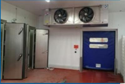
▲ Stainless steel is the material of choice for air coolers operated in fish processing applications as metals are exposed to salt aerosols as well as smoke and are thus much more vulnerable to corrosion.
