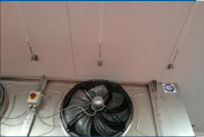
▲ The Güntner air coolers CUBIC Vario, type GGHN, are made of stainless steel and are HACCP-certified by TÜV Süd.
