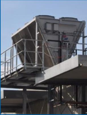
▲ The refrigerant CO<sub>2</sub> is artificially cooled after leaving the Güntner gas cooler V-SHAPE Vario GVD to reduce thermodynamic losses caused by flash gas in the refrigerant lines and to achieve in this way smooth operation of the plant and higher efficiency levels respectively.
