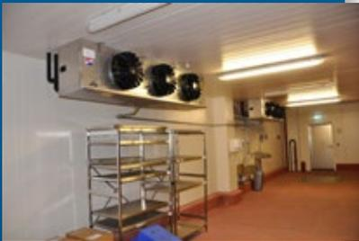
▲ In the processing and order-picking rooms, the Güntner CO<sub>2</sub> evaporators DHF and GHF in stainless steel design with epoxy-coated fins were integrated to prevent corrosion.
