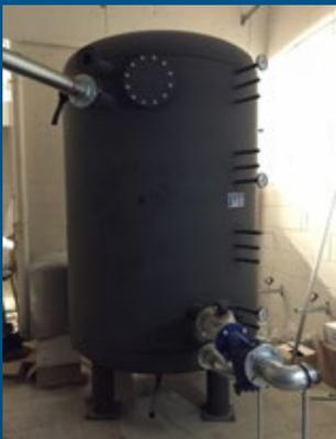
▲ The heat is first stored in a hot water buffer tank with a filling volume of 6,500 l/229.5 ft<sup>3</sup> so that the plant can respond flexibly to heat requirements, allowing to compensate for capacity fluctuations regarding heat recovery.
