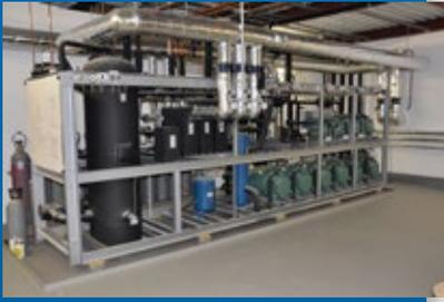
▲ Ten high efficiency compressors that can be used for a wide range of applications are installed in the machinery room and can provide cold for four temperature levels via the evaporating temperature.
