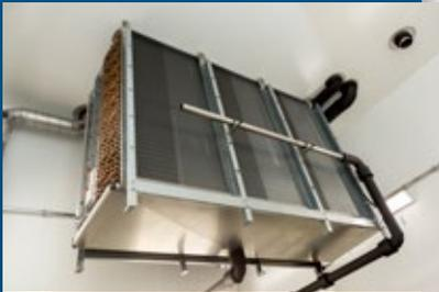
▲ The air coolers are defrosted using warm brine and the process can be enhanced with electric defrosting; as such, the trays are also designed to be heated. As the air coolers have a modular design, both the floor-mounted and ceiling-mounted units were quickly and easily assembled.
