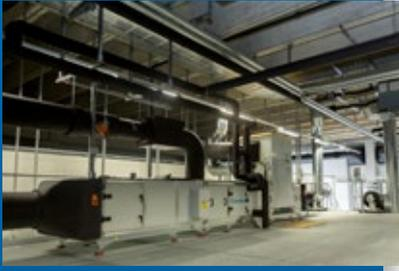
▲ Each ATP climatic chamber is assigned an air conditioning unit which is mounted in an intermediate storey above the test chambers.
