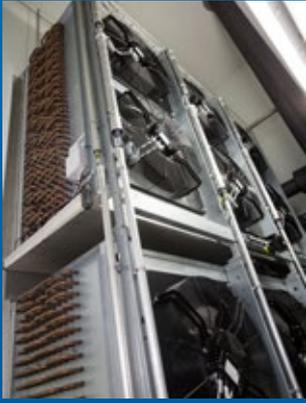
▲ The forced draught fans of the GFN-type Güntner Application BLAST air coolers are mounted behind the climatic chamber.
