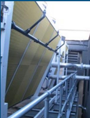
▲ The Güntner dry coolers V-SHAPE Vario GFD are equipped with energy-efficient ebm Axi-Tops to reduce the sound level. The installed HydroSpray system secures the capacity at very high ambient temperature peaks.
