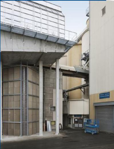
Ten Guntner GCO air heater coils (still without casing in the image) produce hot air for the kiln.
