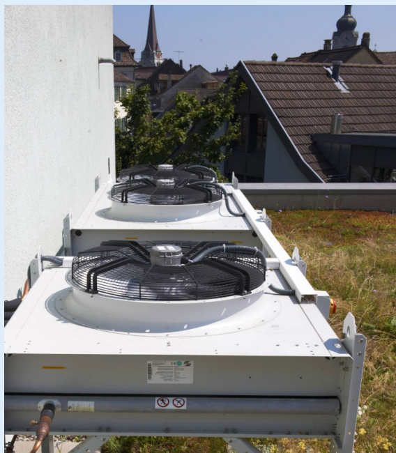
These GVHX condensers are equipped with particularly quiet and energy efficient EC fans.
